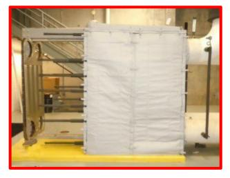
Custom fabricated removable insulation systems provide personnel protection, heat loss & heat gain protection, freeze protection. For heat loss and heat gain, energy savings payback is typically measured in months.
